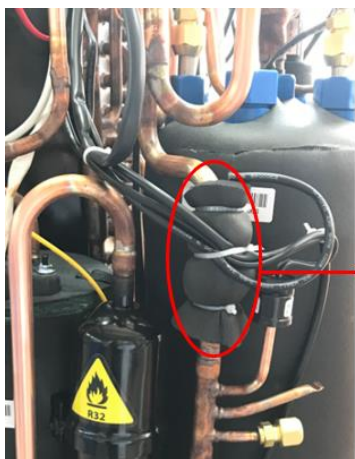
Gas return temp sensor position: near low pressure switch
